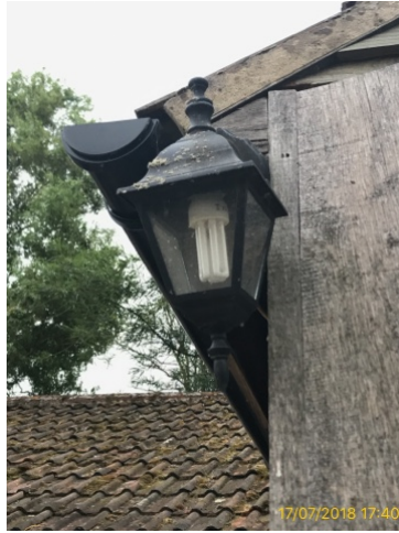
1.5 Lighting (Outside Areas)
