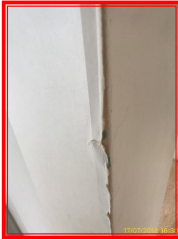
9.3.2 Filled holes / paper lifting around arch .
