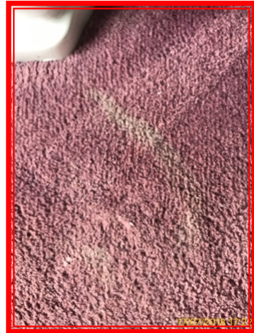
12.10.1 Bleach marks around basin .
