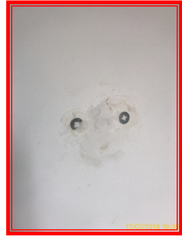
9.3.2 Filled holes / paper lifting around arch .
