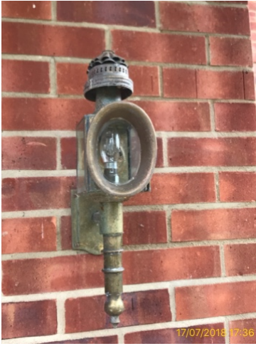
1.5 Lighting (Outside Areas)
