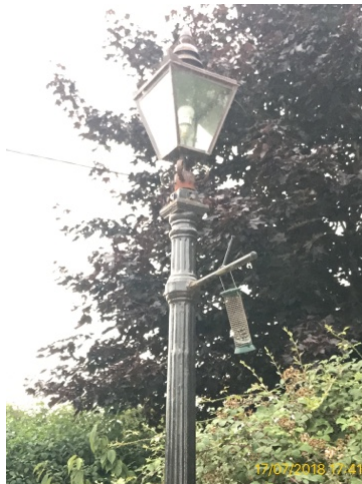
1.5 Lighting (Outside Areas)
