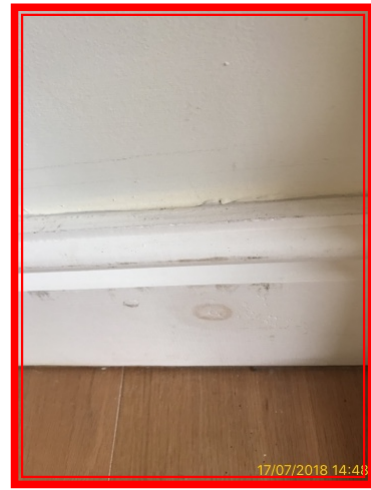
3.11.1 Small chips and scuffs to frames and skirting .
